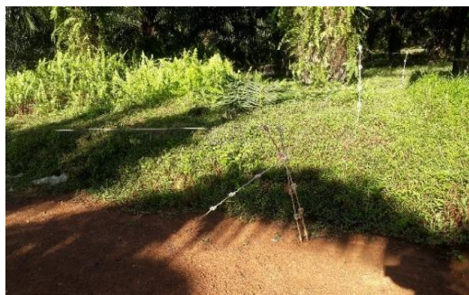
Gambar 36. Pemasangan Electric Fencing
